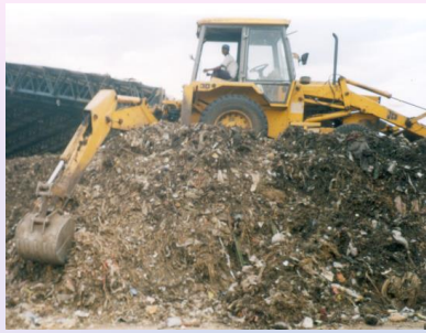
Old Dumped Waste Excavation and Windrowing
